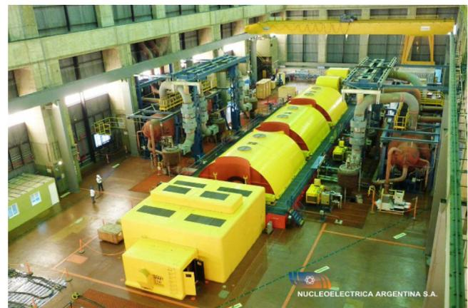
**Fig. 2.** Embalse nuclear power plant turbine generator.
